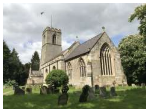
Treswell St John reordering plans underway
